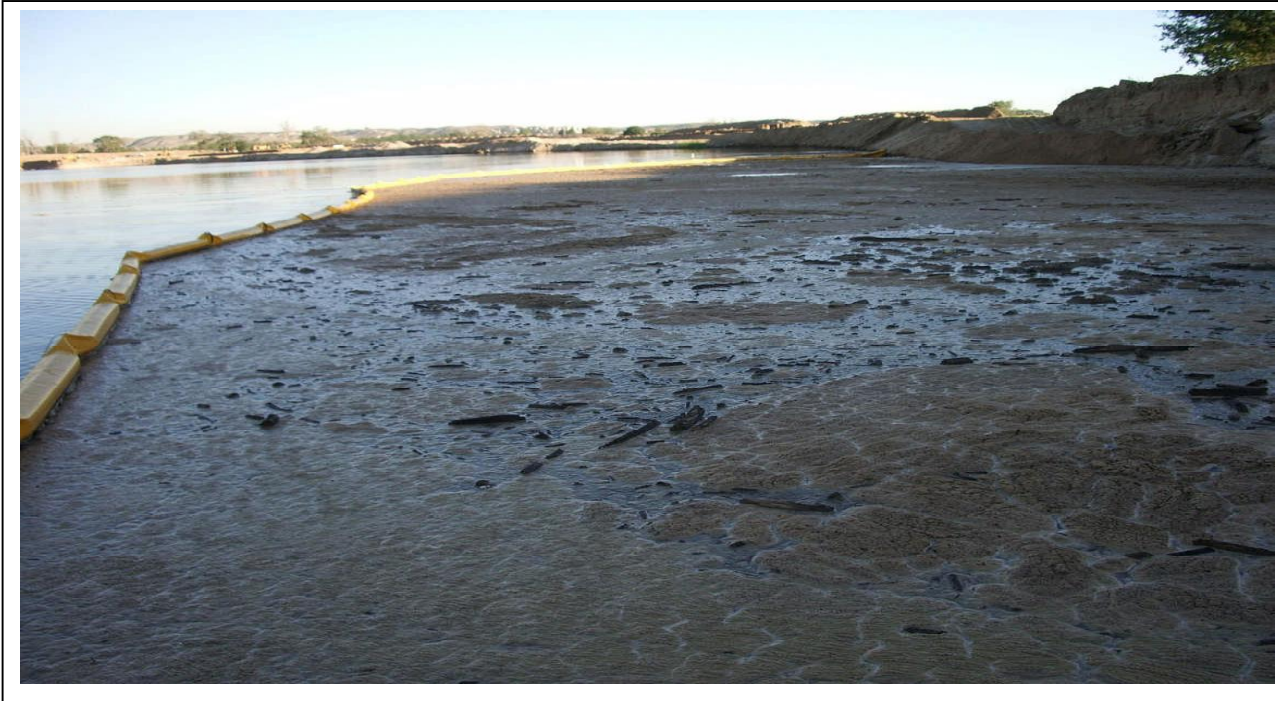
Silt Screen type FCB 75 deployed at a project in Spain.
